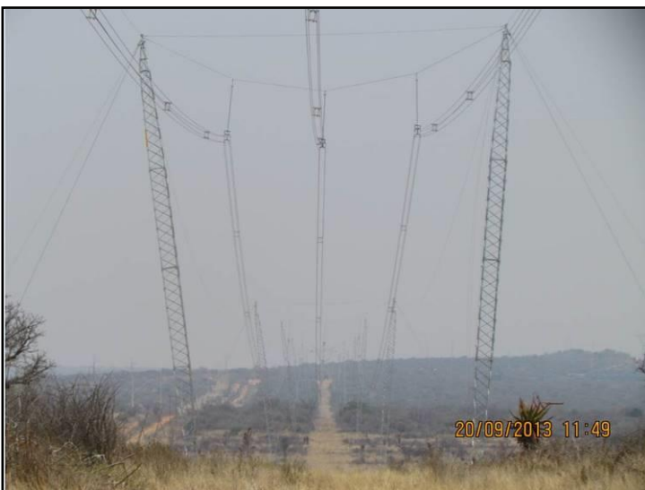
Plate 1: A 529 cross-rope tower
