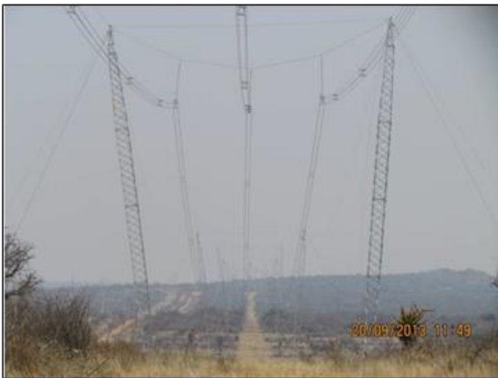
Plate 1: A 529 cross-roped tower
